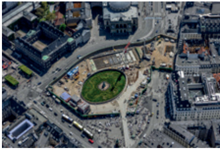
An aerial photo of the construction works for the new Metro station in Copenhagen near the Magasin du Nord. The store is at the top right of the photo
