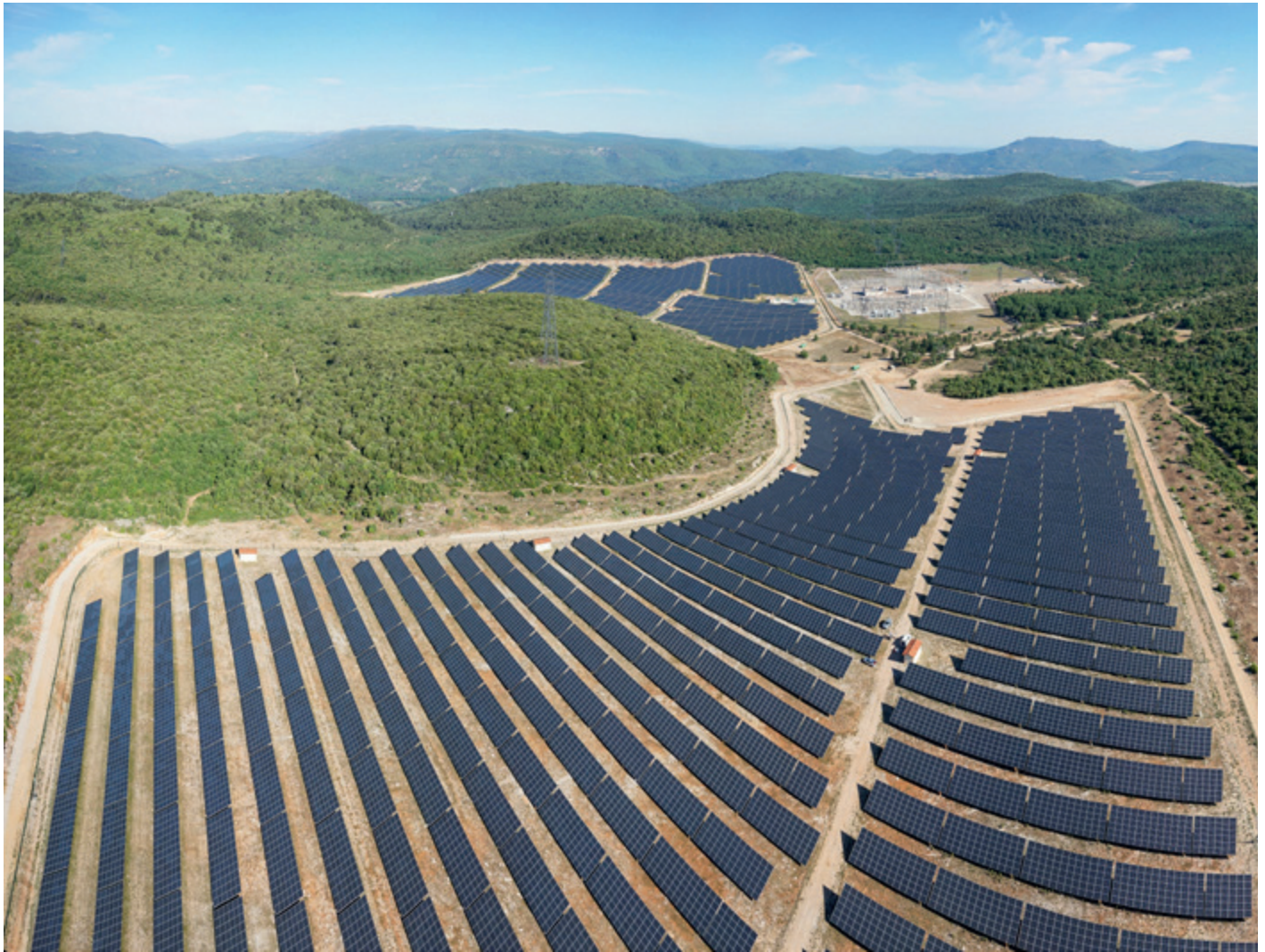
Akua Energy's solar farm covers 30 hectares of land and has more than 75,000 solar modules
