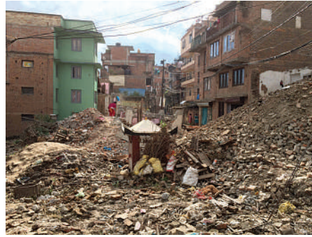
The town of Panga, southwest of Kathmandu, was badly damaged in the earthquakes of spring 2015 (© Randy Braun)
