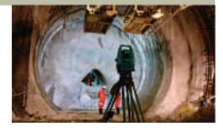
For this task, they used total stations, or optical measuring devices, and GPS, or satellite navigation solutions from Leica Geosystems. There was no major delay during construction time, and the tunnel was inaugurated on June 1st as planned.
