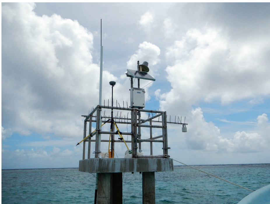
A GNSS receiver set up on a benchmark point on the new instrument platform. Long-session GNSS observations enable researchers to establish precise control and monitor any motion of the platform.
