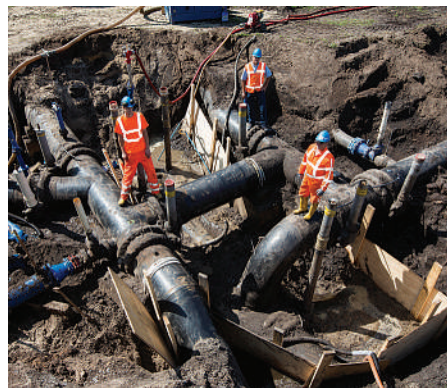
Water pipe maintenance (courtesy of Oasen)
