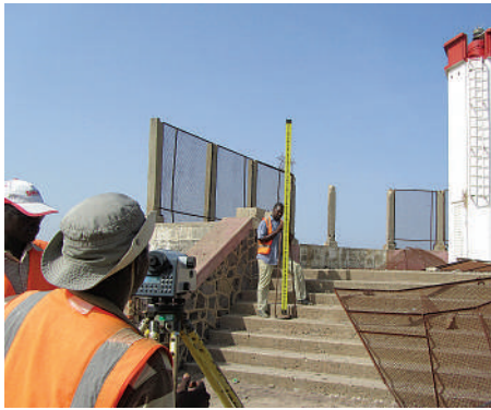
Altimetry tie of the Dakar recording tide gauge (Senegal) ©IGN
