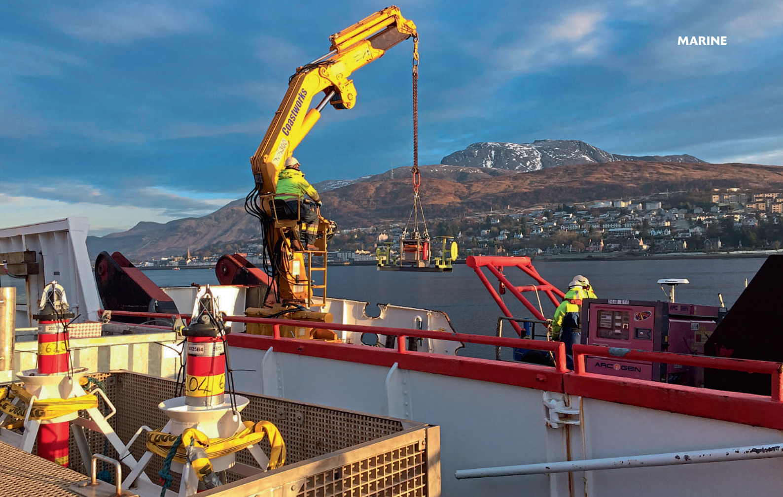
Lowering subsea structure 'reference frame' onto deployment vessel, complete with vertical and horizontal flanges © DOF Subsea
