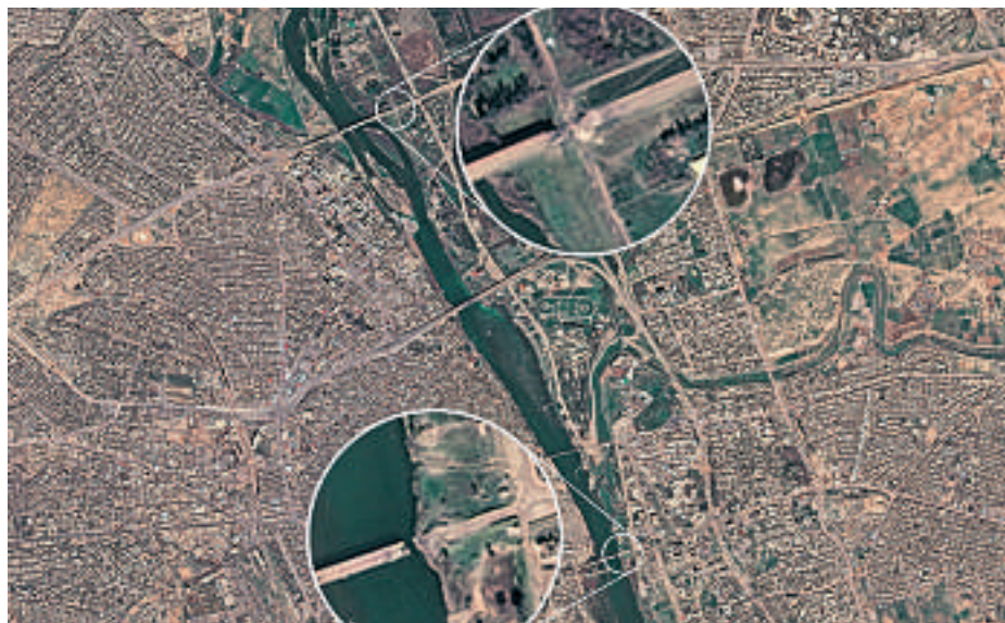
Figure 1. Deimos-2 image of the city of Mosul showing 2 of the 5 badly damaged bridges. Upper zoom in: Al-Shohada Bridge; lower zoom in: Al-Jamhuriya Bridge. Image captured on March 10 2017
