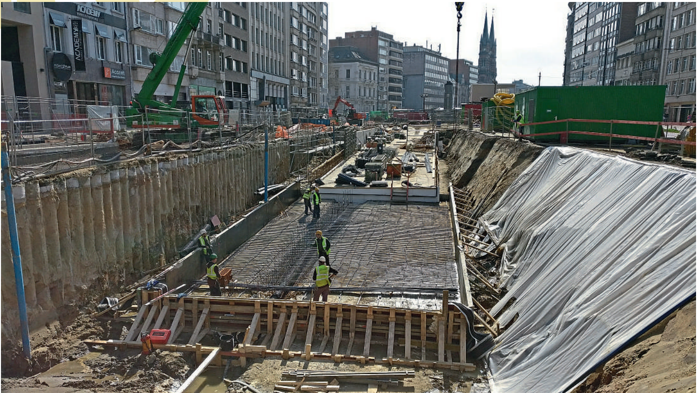
Building the tunnel floor of the first of four road tunnels. This is the southwestern tunnel connecting the Frankrijklei with the underground Opera station and car park. Just a couple of hours before pouring the concrete. © Noorderlijn
