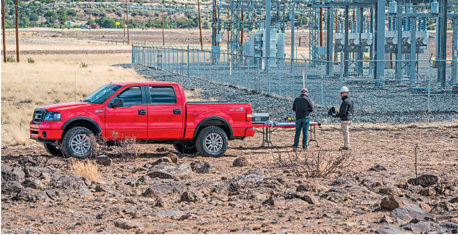
UAVs allow sites to be monitored without risking the health and safety of surveyors
