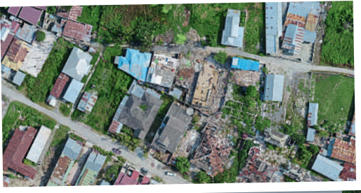
Aerial orthomosaic of an area damaged by the earthquake
