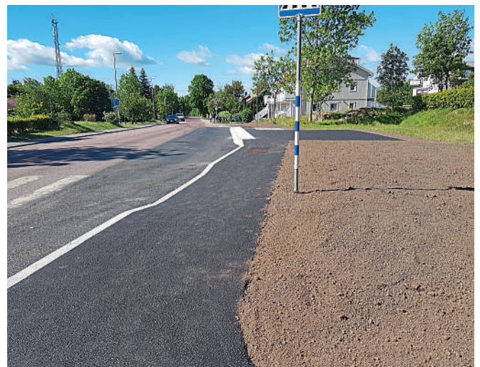
A bus stop in Uppsala County before and after updating. Safety improvements include wider lay-bys and improved pedestrian access. A new shelter and bicycle parking would be installed later
