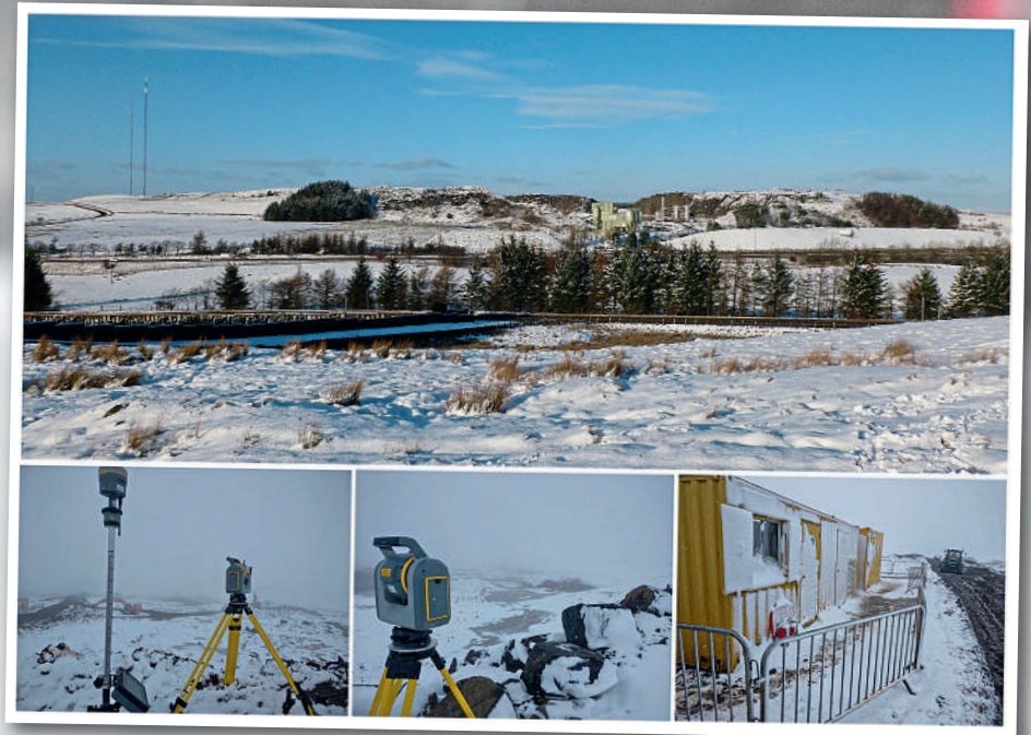
Top: Storm Emma blankets Duntilland Quarry in heavy snow. Photo: cc-by-sa/2.0 - © Alan O'Dowd. Lower left: SX10 and R10 at the quarry. Lower Centre: The SX10 collects scanning data during the blizzard. Tri-Tech used polygon-defined scanning regions to reduce time in the field. Lower right: Blizzard conditions prevented the use of UAVs
