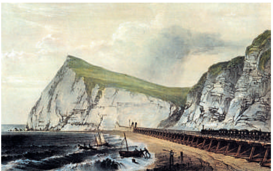
Fig.1: The original timber trestle viaduct (pictured) has since been buried up to the railway trackbed
