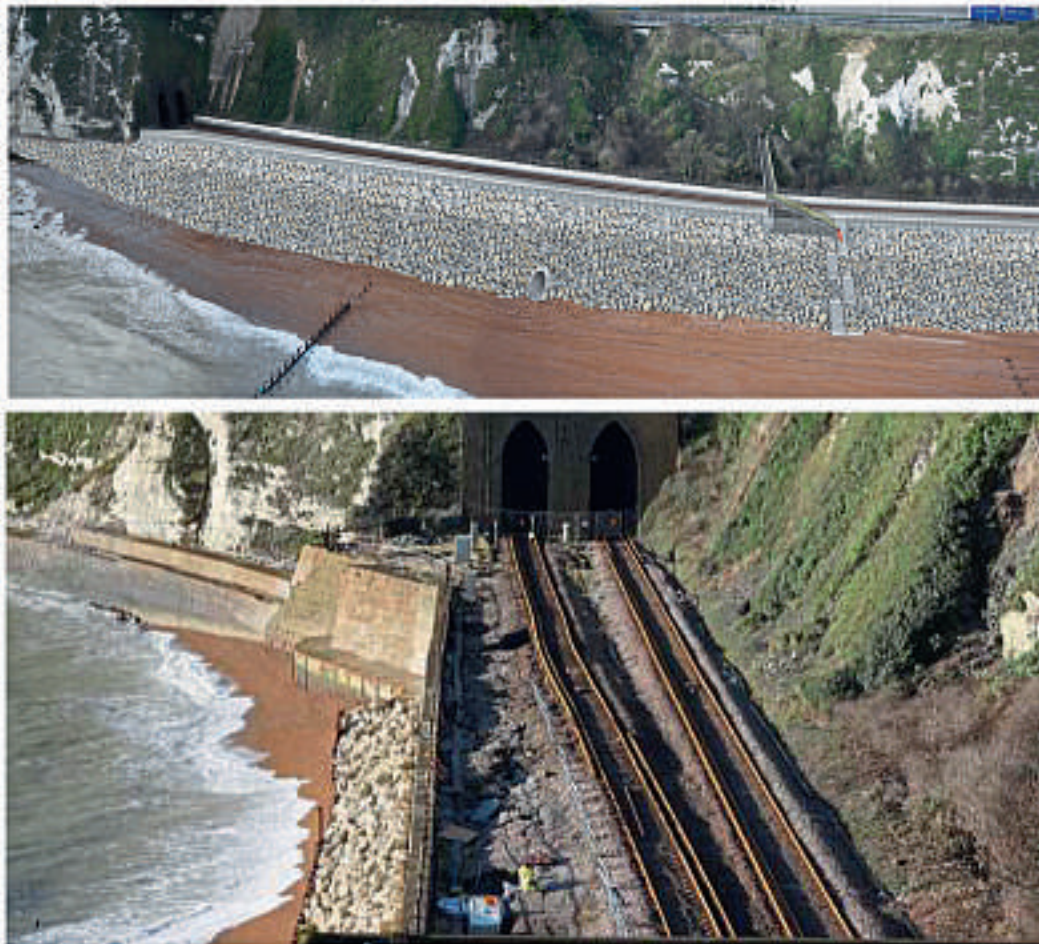
Fig.3: The reinforced Dover Sea Wall and reinstated rail track
